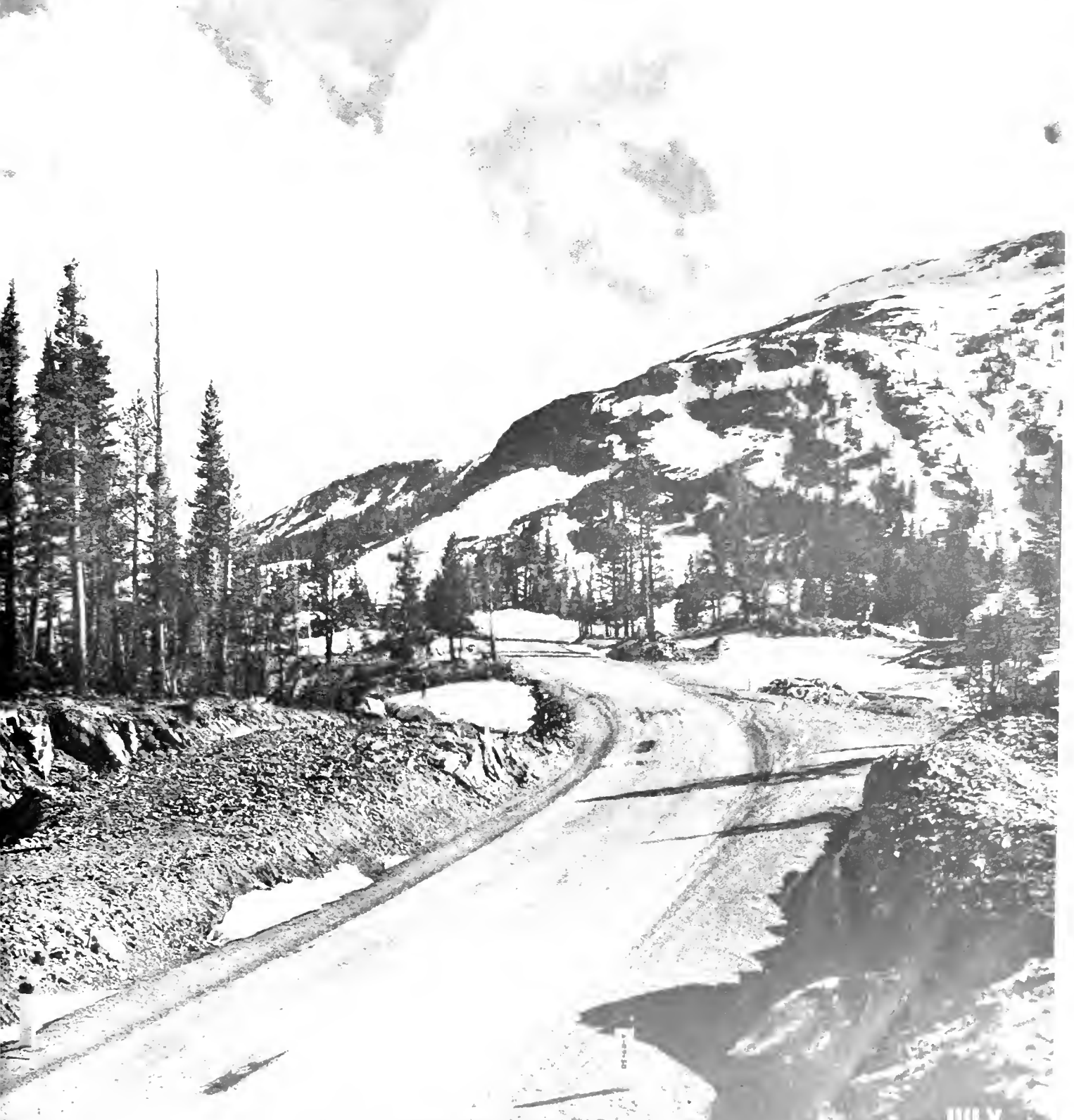
VIEW OF SECTION OF NEW TIOGA PASS HIGHWAY LOOKING WESTERLY FROM A POINT BETWEEN LAKE ELLERY IN MONO COUNTY AND THE TIOGA PASS EASTERLY ENTRANCE TO YOSEMITE VALLEY (SEE ARTICLE IN THIS ISSUE)
